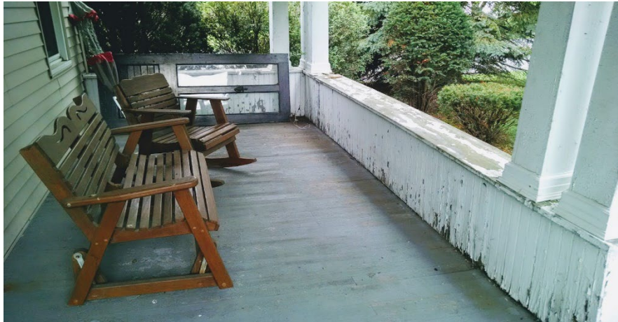
Photo 1 – Porch Before Renovation
