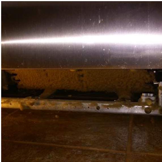
The image above (bonus point if you identified it) is a dust and lint caked coil on the bottom of a late model refrigerator. The image below is after cleaning.
